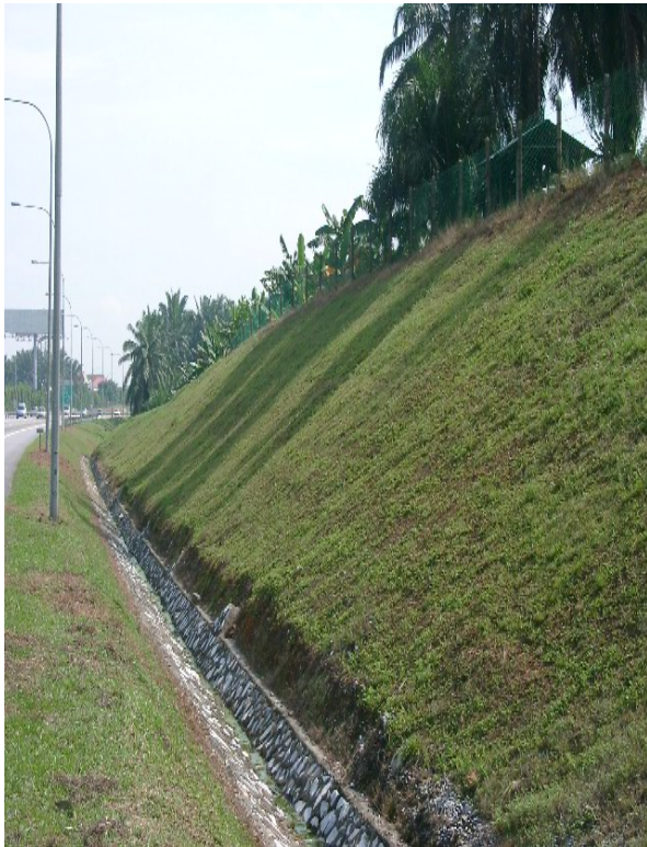
(a) V-drain along Toe of Slope
